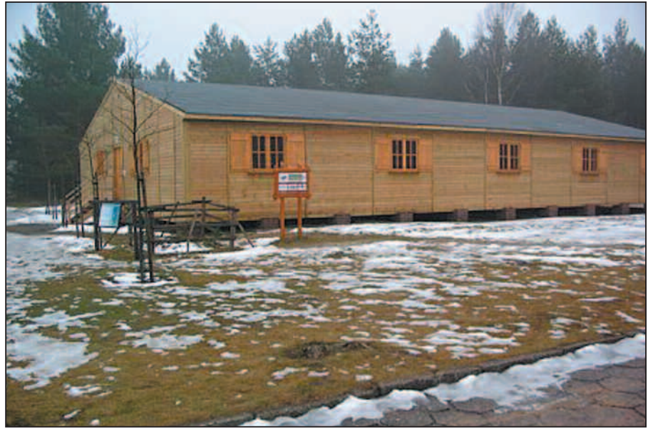
An RAF Hut, Stalag Luft III
